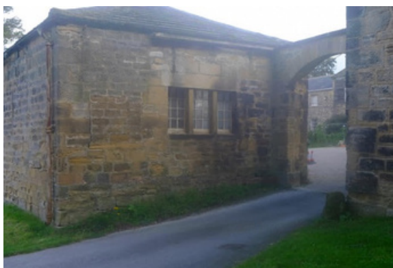
Photograph from planning application
