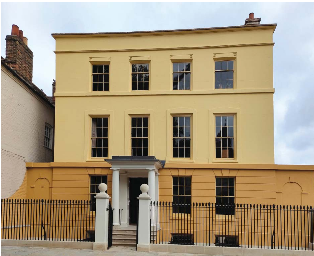
Chatham House after the restoration project was complete in September 2022. (Credit: Medway Council)
