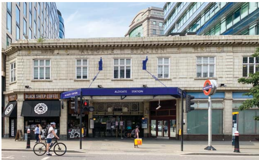
The 1926 frontage to the unlisted Aldgate Underground Station (Credit: SAVE Britain's Heritage)
