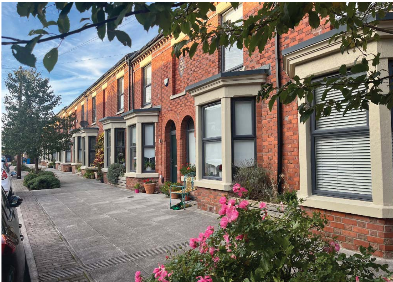
“Two-into-One” restorations of the terraces of Voelas Street, Liverpool 8, pictured exactly 10 years after SAVE forced a public inquiry into their managed decline and demolition. (Credit: Jonathan Brown)
