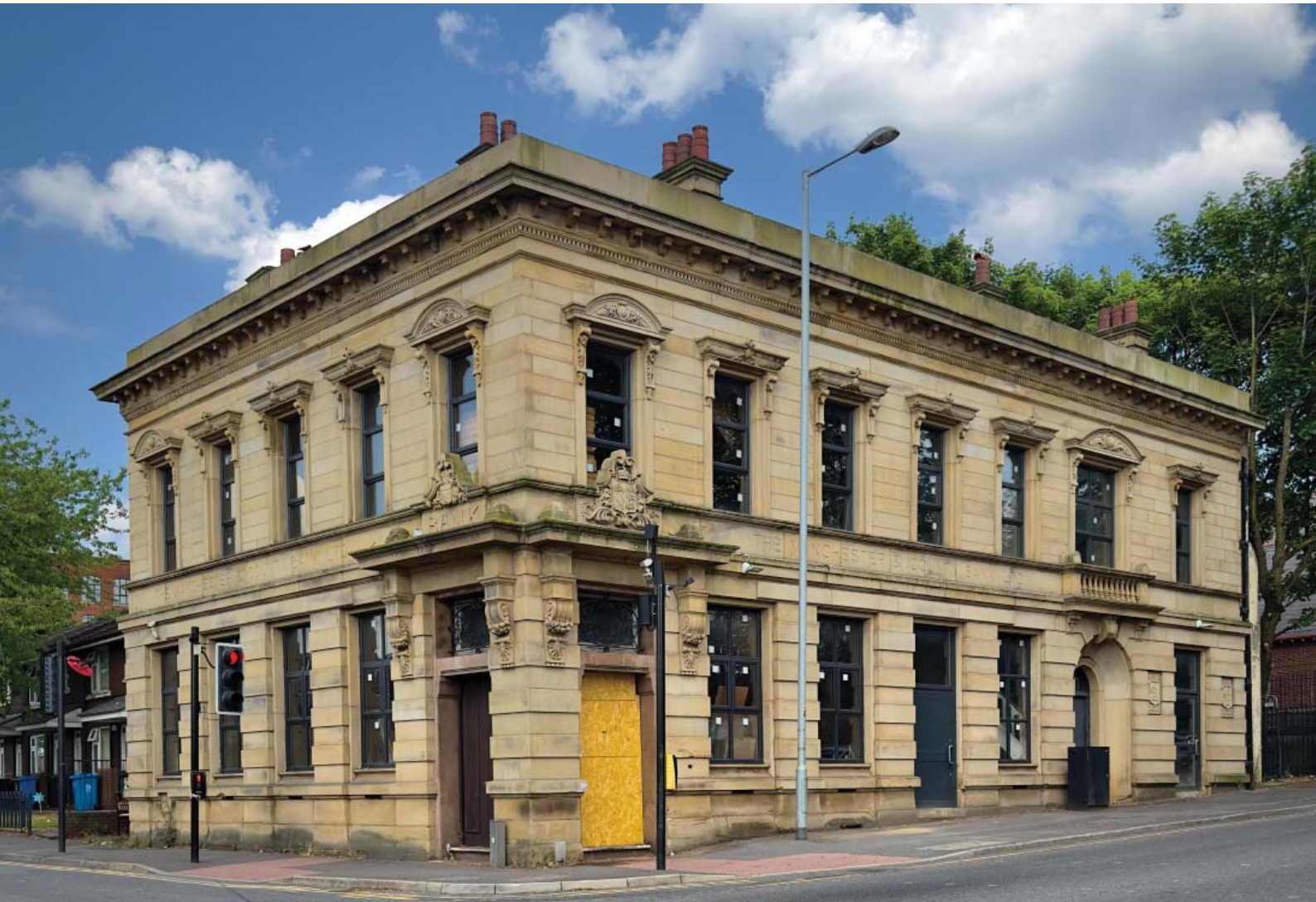
Below: Former Manchester & County Bank, corner of Middleton and Featherstall Roads, Oldham (Credit: Mark Watson)
