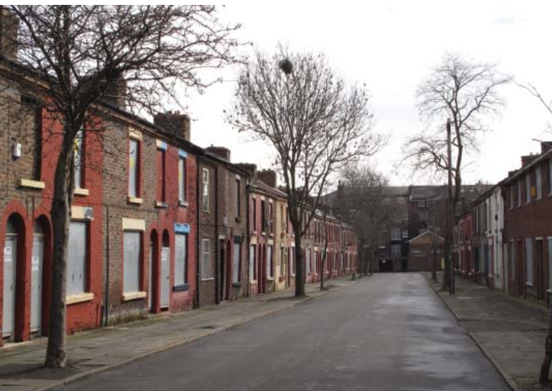
Condemned: hundreds of attractive homes in Toxteth were set to be bulldozed before SAVE stepped in. (Credit: Jonathan Brown)
