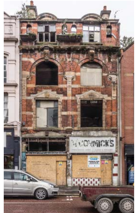
The now lost 107 North Street in 2015. Credit: William Murphy.
